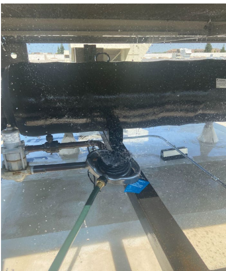
Figure 24: Red Bluff Site with Sprinkler Under the Air-cooled Condenser
