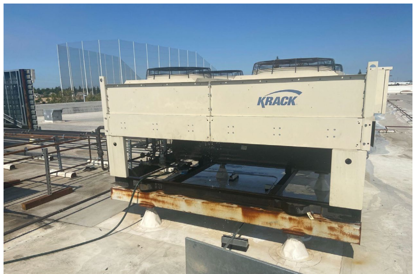
Figure 24: Red Bluff Site with Sprinkler Under the Air-cooled Condenser
