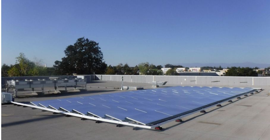
Figure 11: Photo of the SkyCool Array at Red Bluff Site
