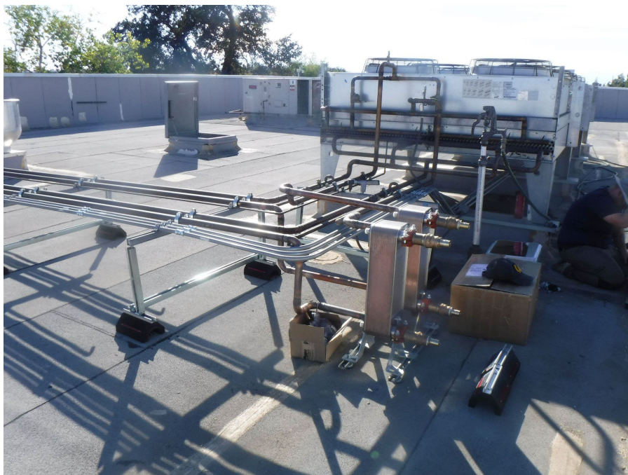
Figure 10: Photo of SkyCool Heat Exchangers Being Installed
