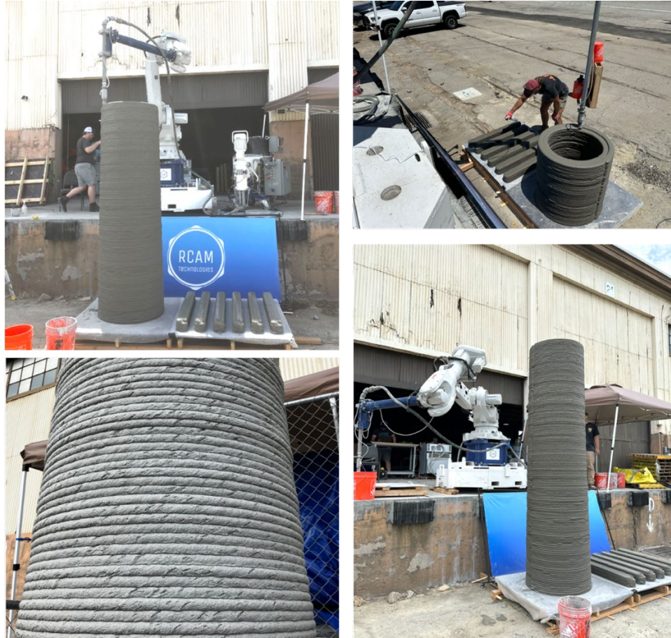
Figure 24. Outdoor Printing of the 3-m-tall Reinforced Tower
