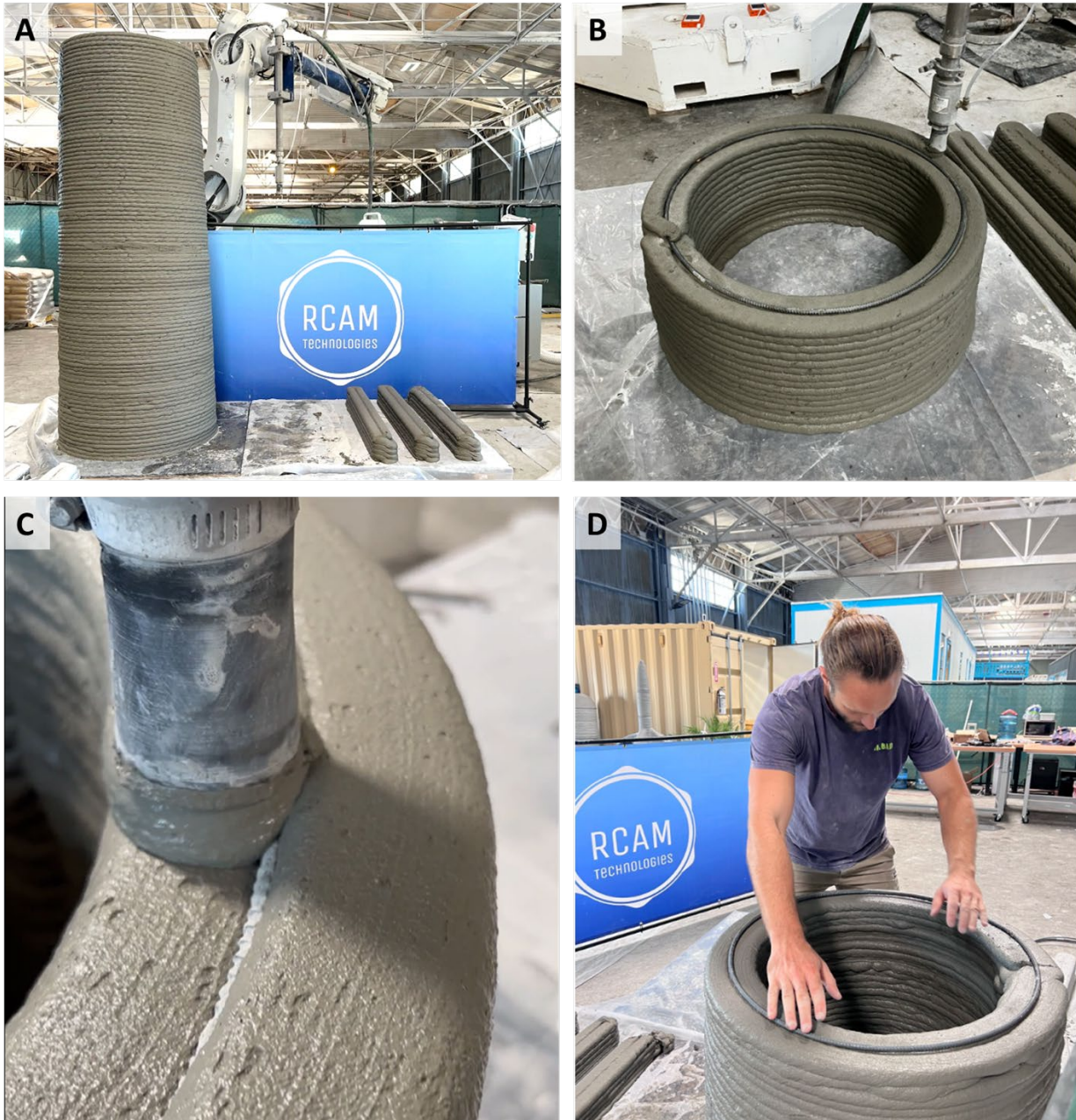
(A) Printed 2-meter tower prototype and sample beams, (B) top view of the double wall print path over reinforcement hoop (C) close-up of printing over reinforcement, and (D) laying a reinforcement hoop.
