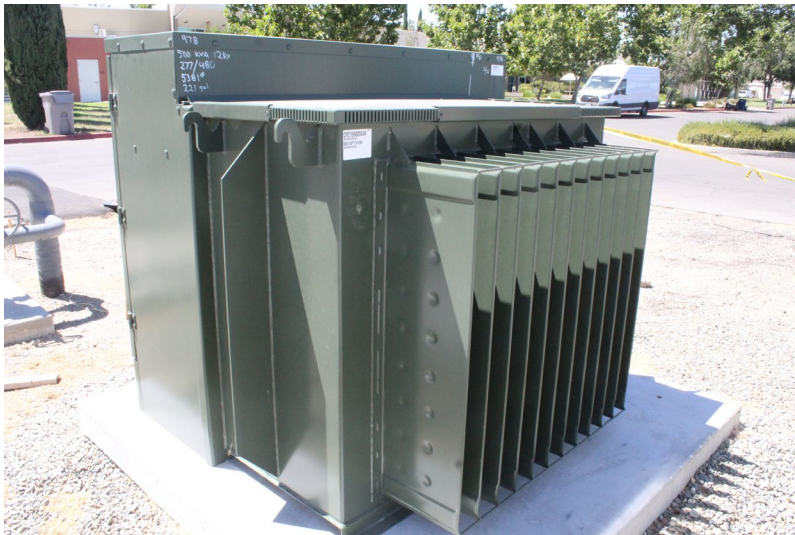
Figure 13 shows rear view of large green SMUD transformer in place on its concrete pad. At front are the large fins to facilitate heat rejection.
