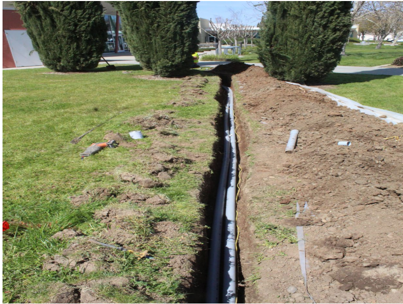
Figure 12 shows electrical trench cut through grass field behind one of the Administration Buildings. Two light gray electrical conduits are in place at the bottom of the trench.
