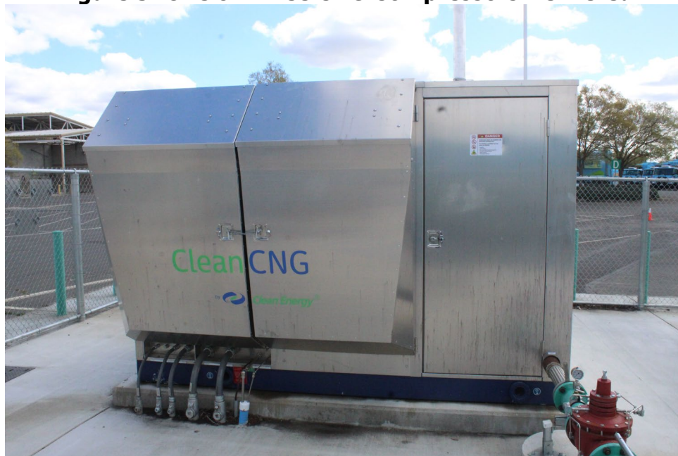
Figure 5: One of Three CNG Compressors Delivered
