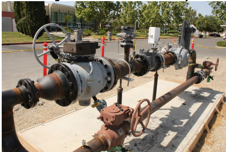
Figure 11: Gas meter Assembly
