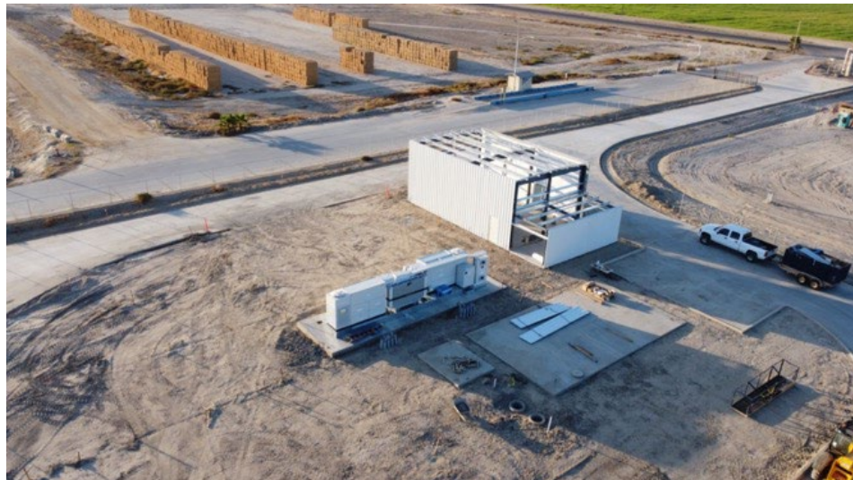
Figure 8: Electrical Room and Rectifier
