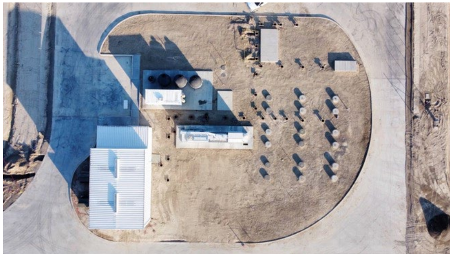
Figure 10: Electrolyzer, Compressor and Chiller Foundations
