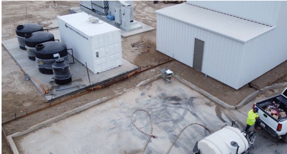
Figure 9: Water Treatment Plant Installation
