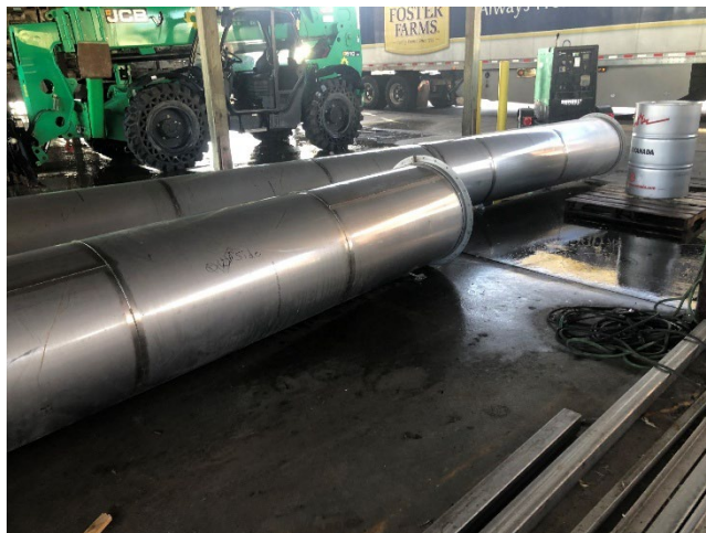
Figure B-21: Livingston Old Piping
