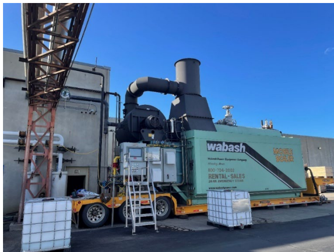
Figure 8: Rental Boiler in Operating Position
