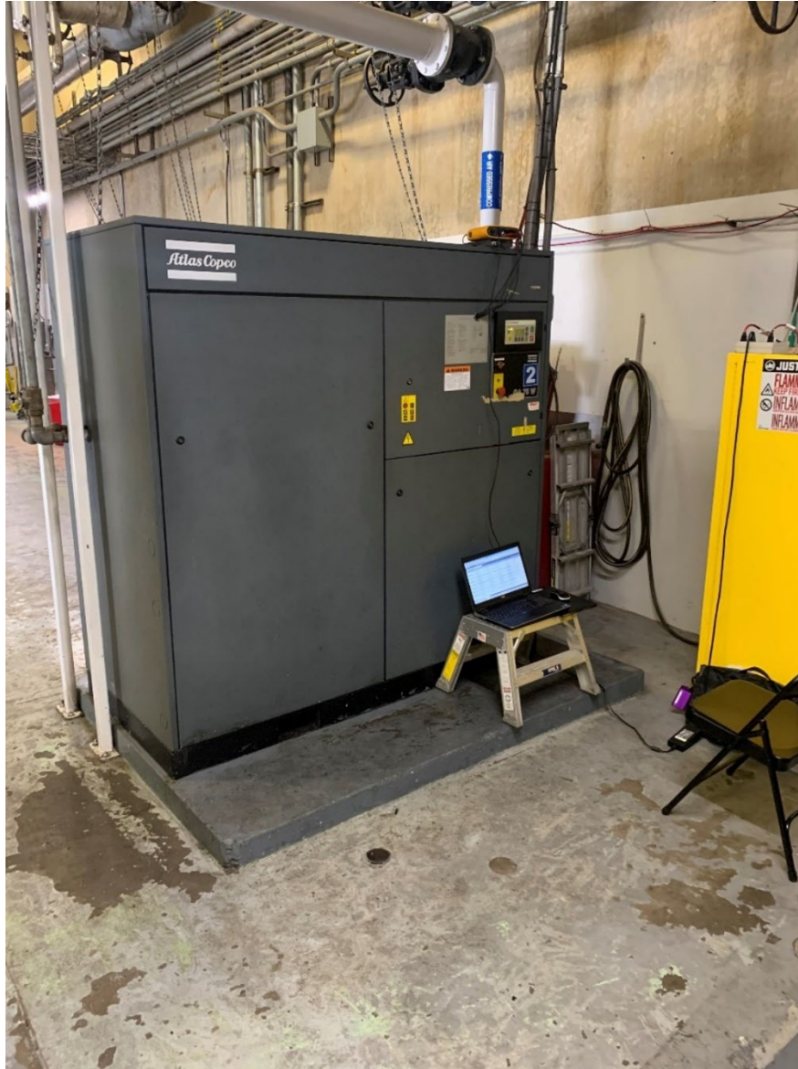
Figure 5: Pre-install Measurement of Old Air Compressor
