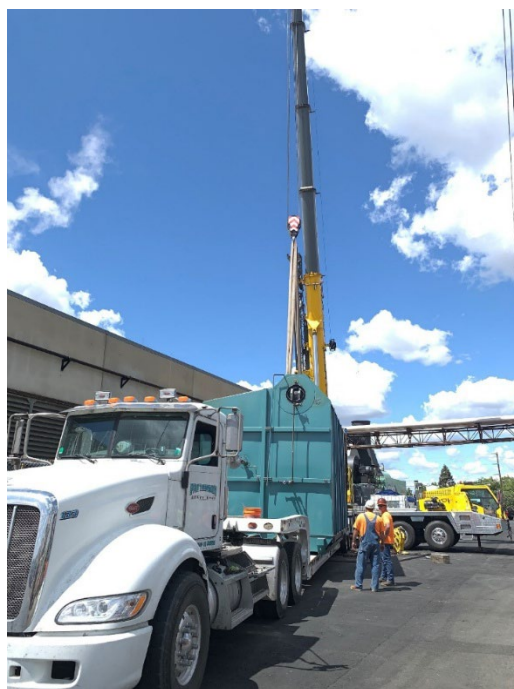
Figure 9: Crane Hauling Away Old Boiler #1
