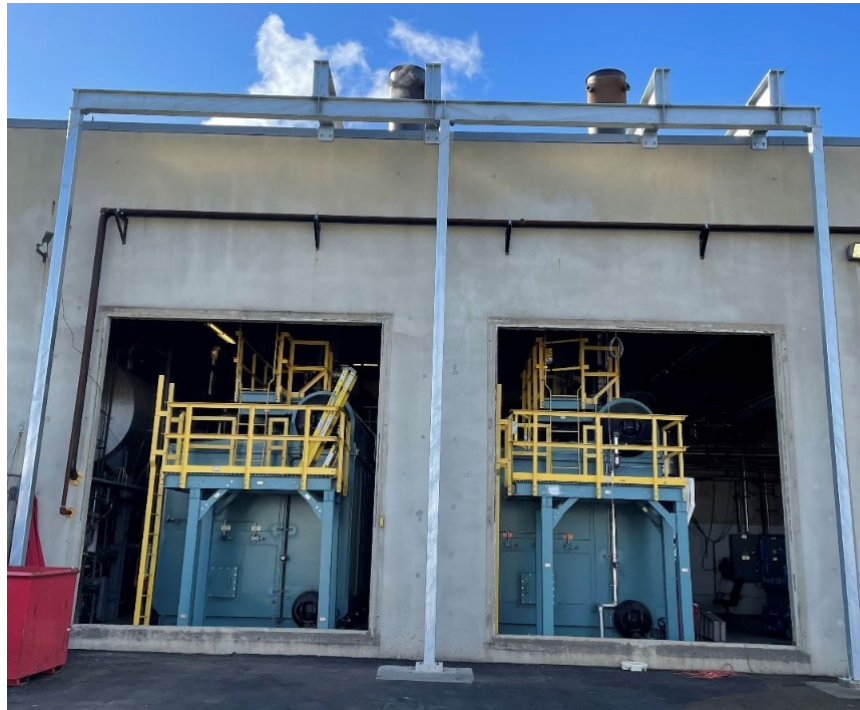
The exterior steel structure that was built to support roof mounted boiler equipment. Also shown is the rear of the newly installed boilers.
