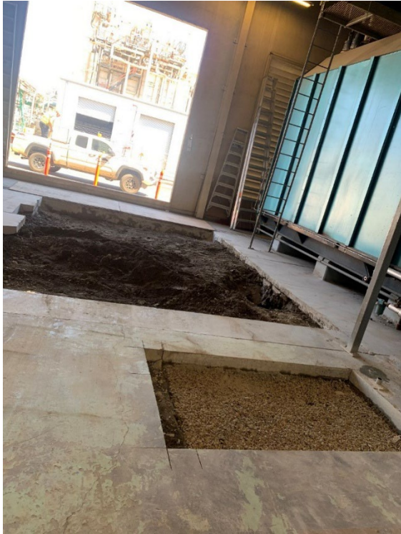
Figure 10: Foundation Prep for New Boiler #1
