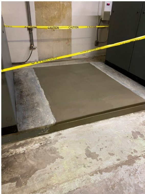
The concrete modification to the pedestal the new air compressor sits on.
