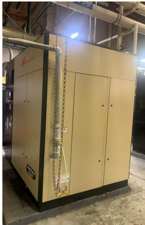
The operator side of the new 200 HP air compressor.
