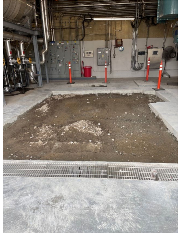
Figure 11: Foundation Prep for New Boiler #2
