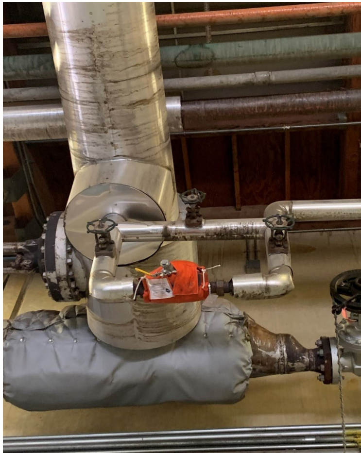
An installed steam trap with the manufacturer-supplied insulated jacket.
