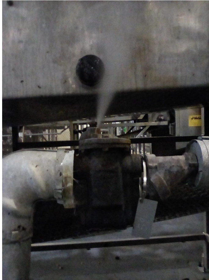
Trap 59 of 175 showing the leak in the trap allowing steam to escape.
