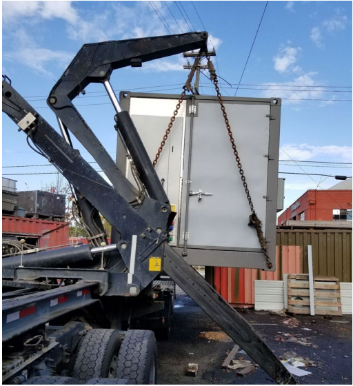
Figure 21: Side-Lifter Moving MG1003; MG1003 Initial Installation at GWRV
