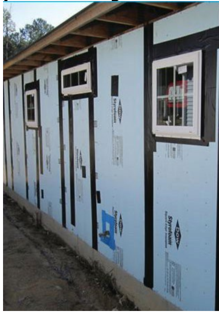
Figure 3-9: Properly Installed Rigid Insulation With Sealant Tape
