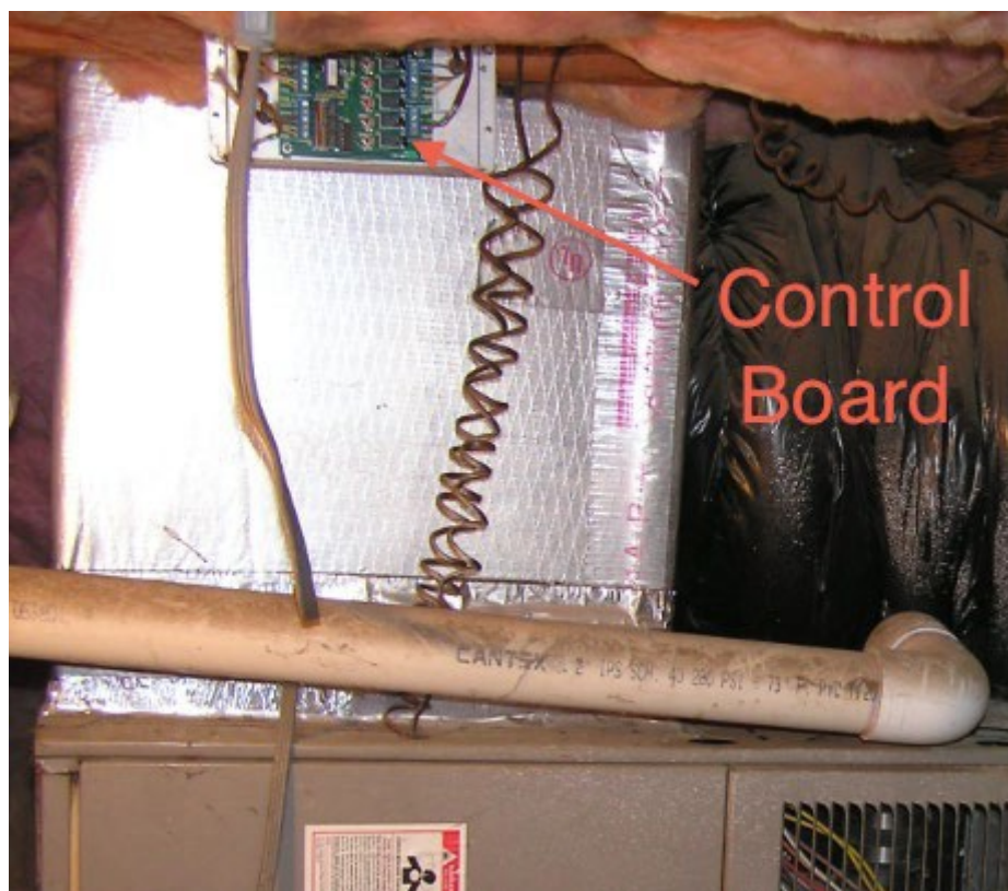
Figure C-6: Photo of a Duct-Mounted Control Board
