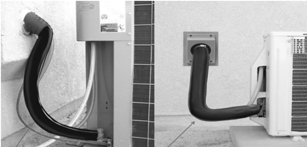
Figure 4-16: Refrigerant Line Insulation
