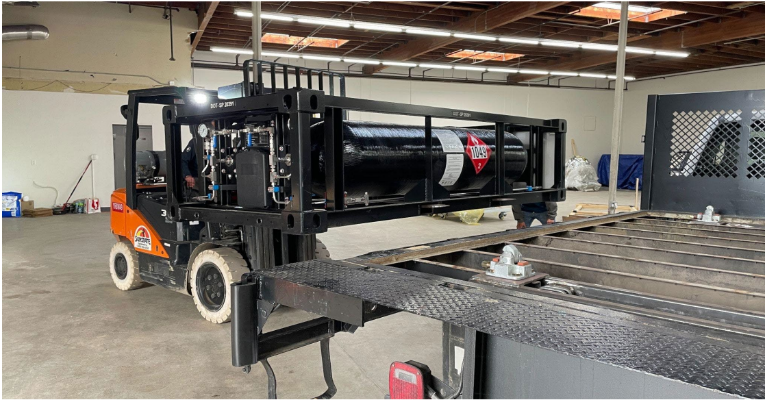
Figure 13: Hydrogen Tank Array Installation
