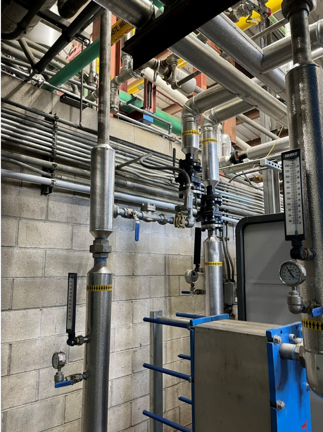
Figure C-1: Heat Exchanger Piping Tie-Ins
