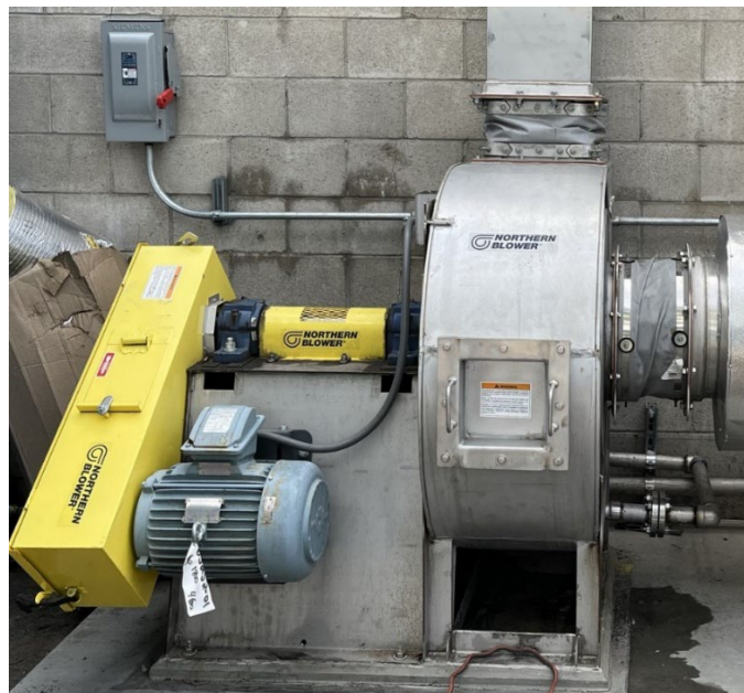
Figure 4: Industrial Centrifugal Fan
