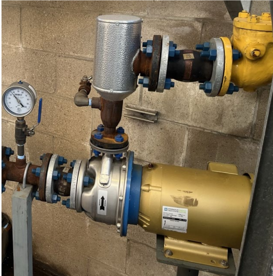
Figure 5: Centrifugal Close-Coupled Pump
