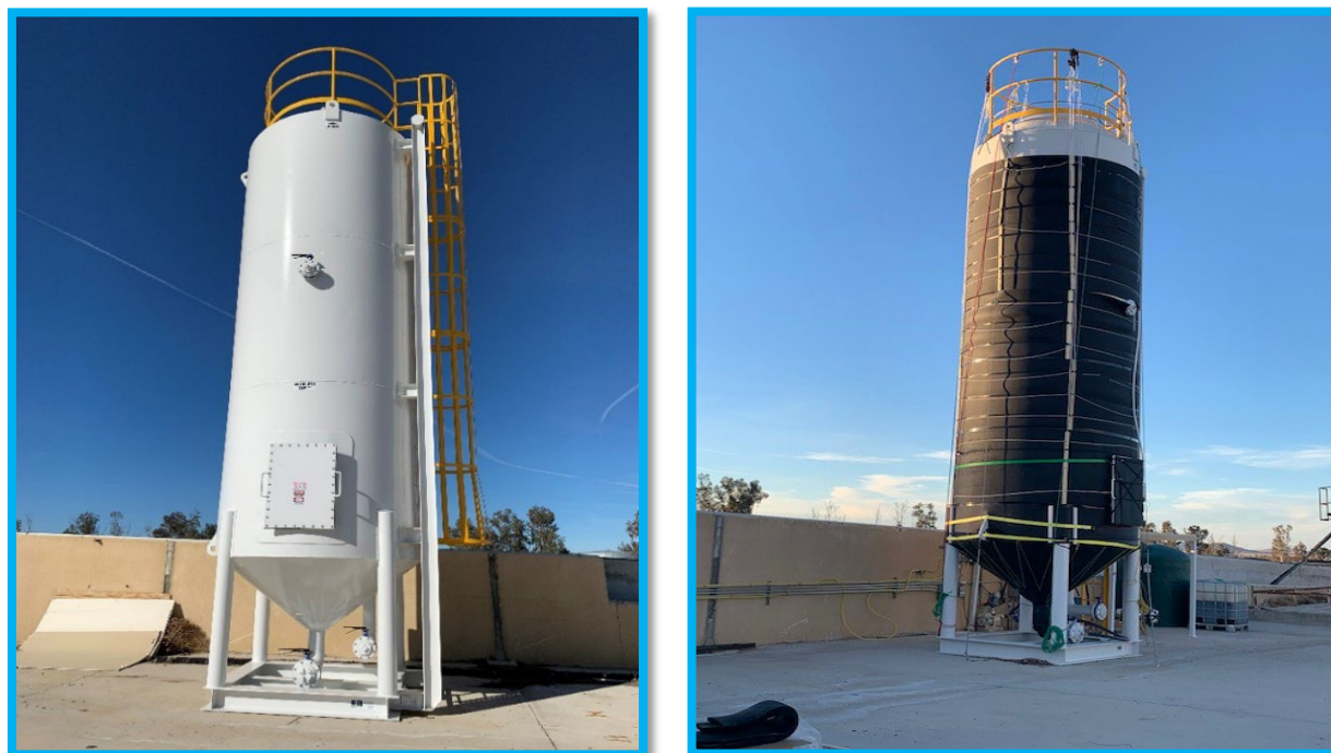
Figure 9: Digester Tank as delivered (left) and with exterior insulation (right)
