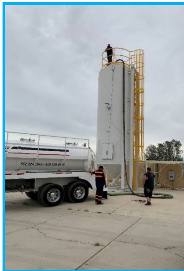
Figure 5: Tank supplying process water and organic substrates onsite
