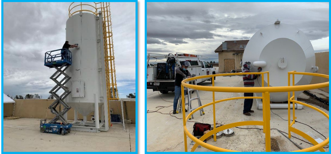
Figure 3: AD tank installation: side ladder with cage (left) & top handrail (right)
