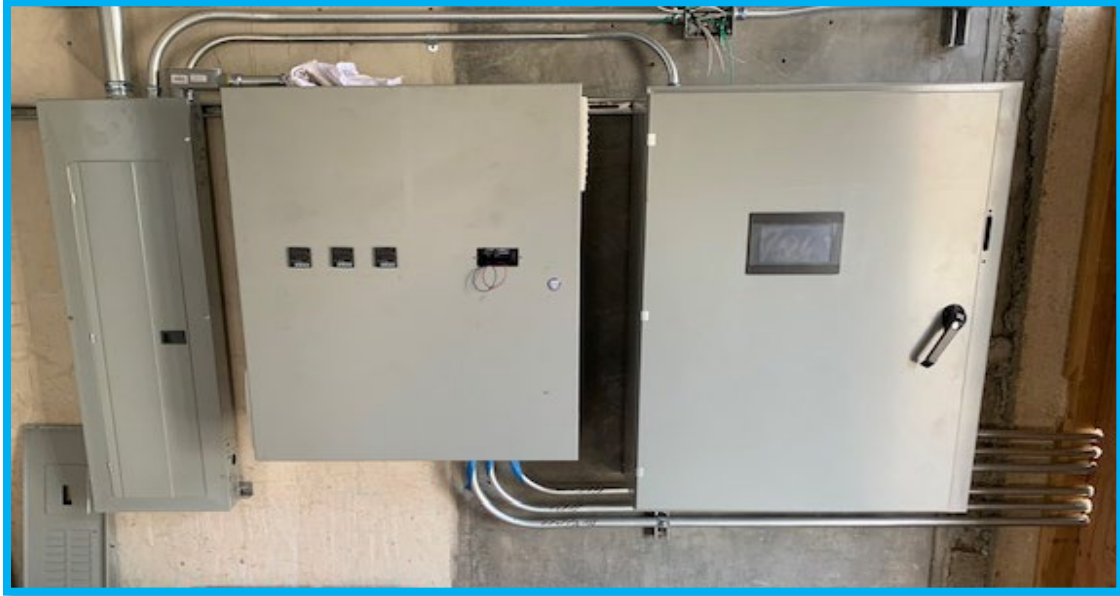
Figure 6: Main Electrical Panels
