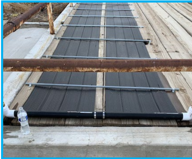
Figure 8: Solar heating blankets for digester heating
