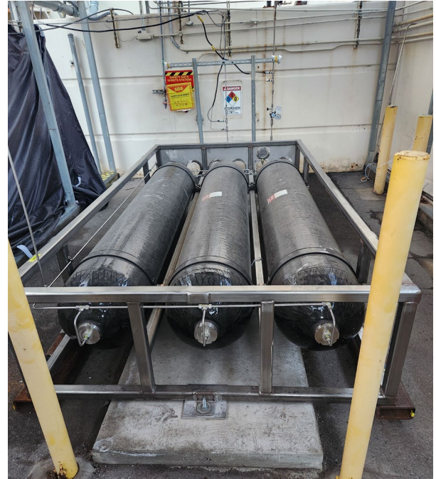
Figure 8: Alkaline Electrolyzer and High-Pressure Hydrogen Storage
