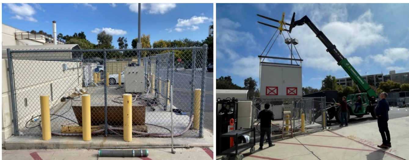
Figure 7: Pre-Existing Pad and Installation of Containerized Alkaline Electrolyzer
