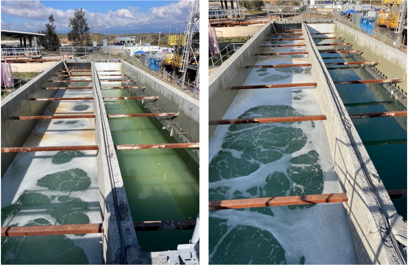
Operation of BDP Wastewater treatment system.
