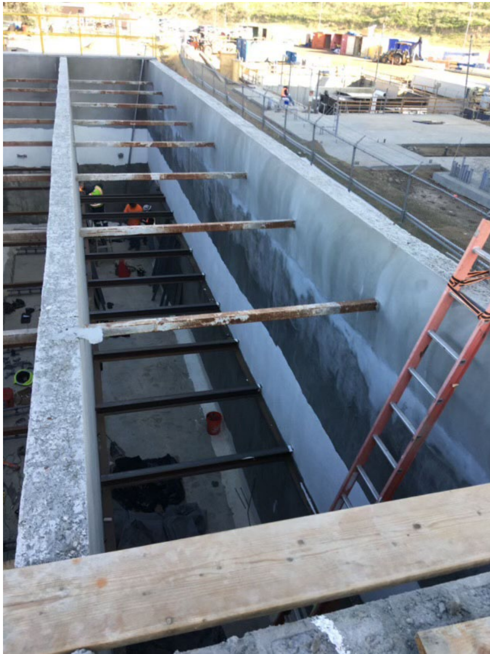
Constructing the raised walls of the BDP biological basin.
