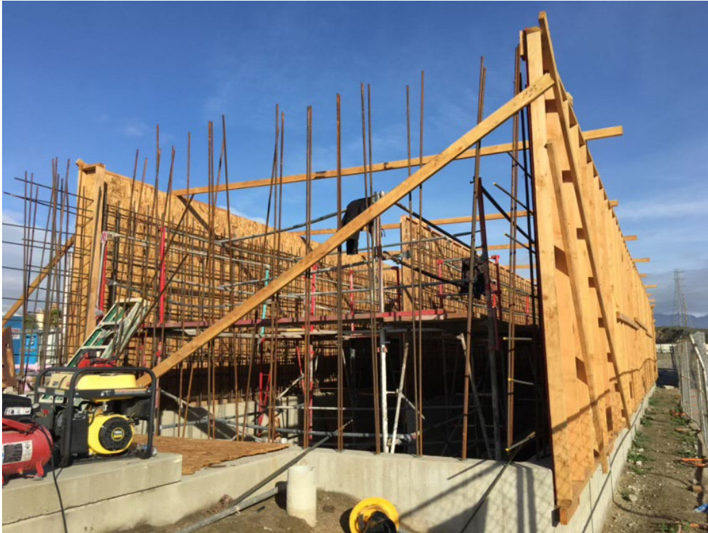
Figure A-2: Construction of BDP Biological Drain
