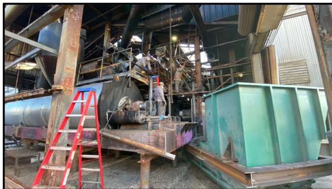
Figure 7: Dismantling the Old Hopper
