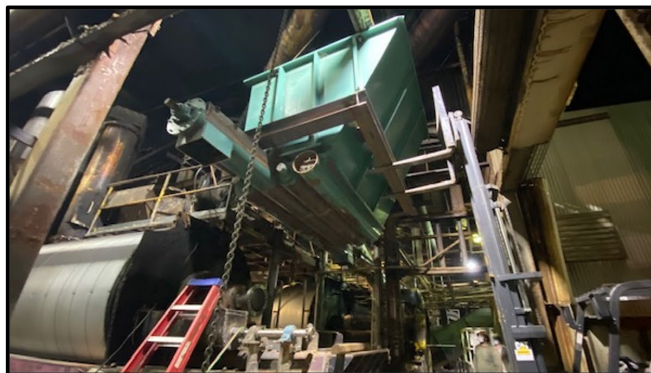
Figure 7: Dismantling the Old Hopper
