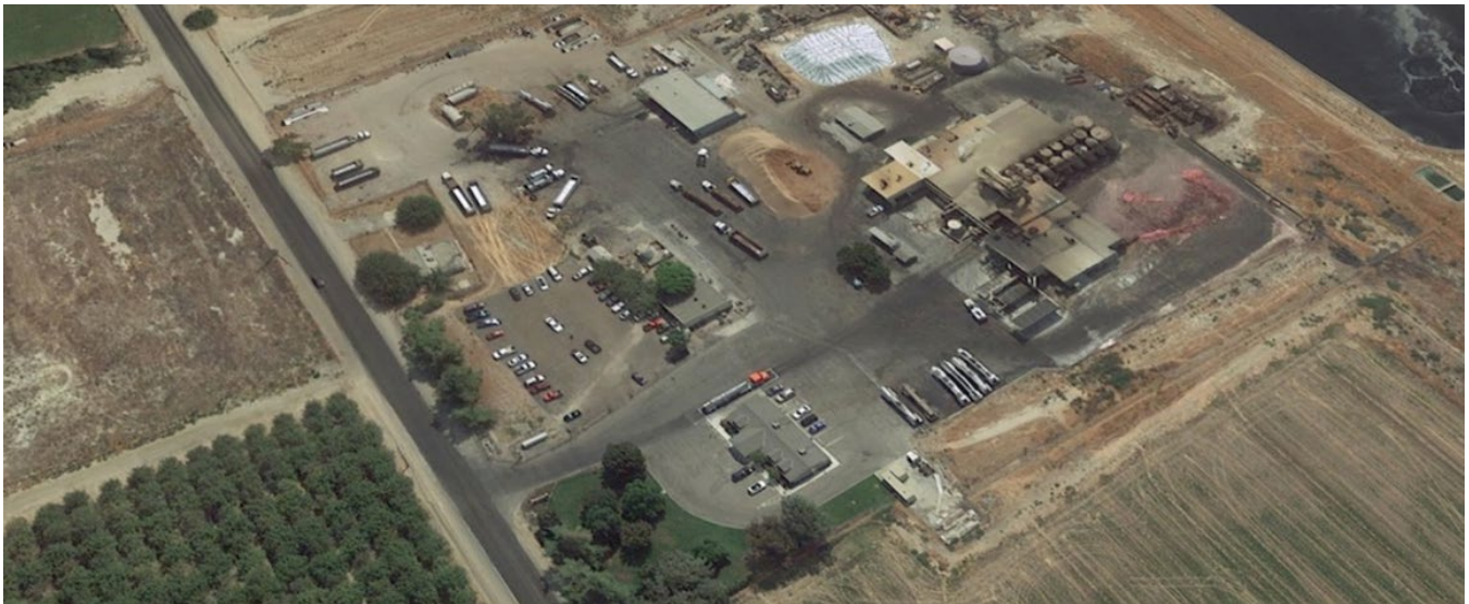
Figure 1: Overview of the Baker Commodities, Inc. Facility
