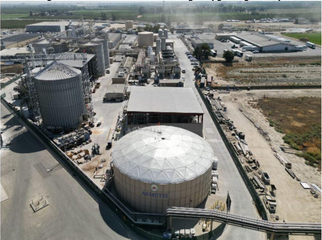
Figure 14: Overview of Aemetis Biogas Upgrading Facility
