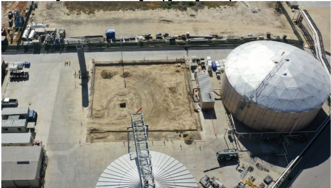
Figure 9: Aemetis Biogas Upgrading Facility Foundation
