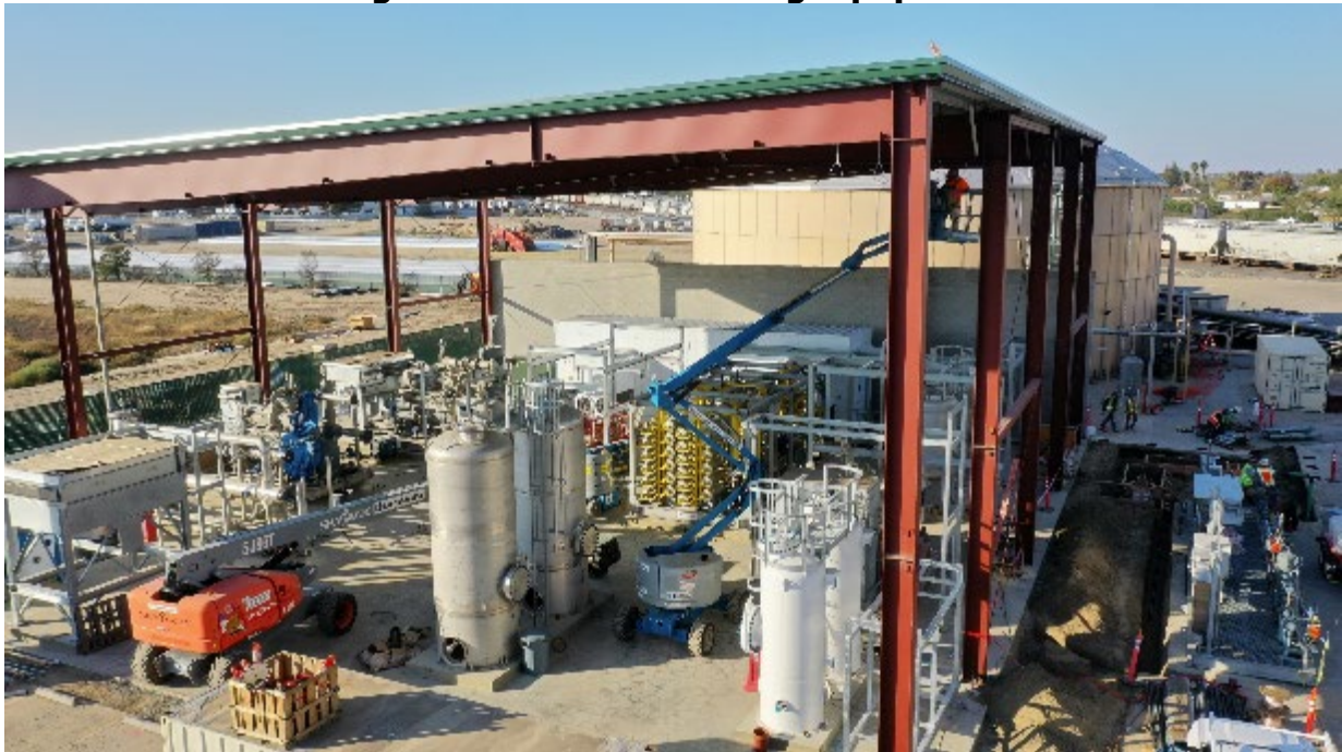
Figure 12: Aemetis Setting Equipment
