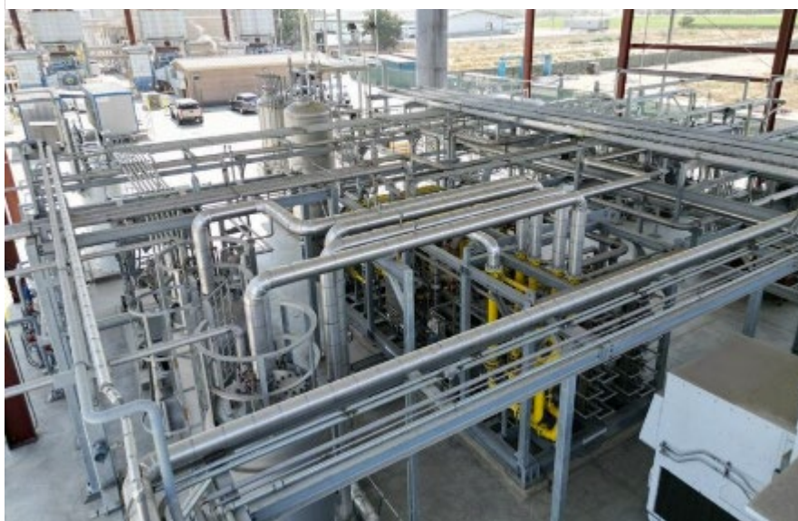
Figure 4: Top View of Aemetis Facility
