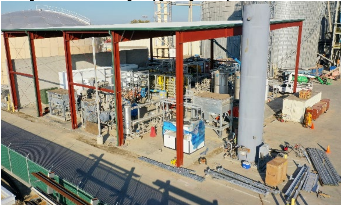
Figure 11: Aemetis Biogas Upgrading Facility under construction
