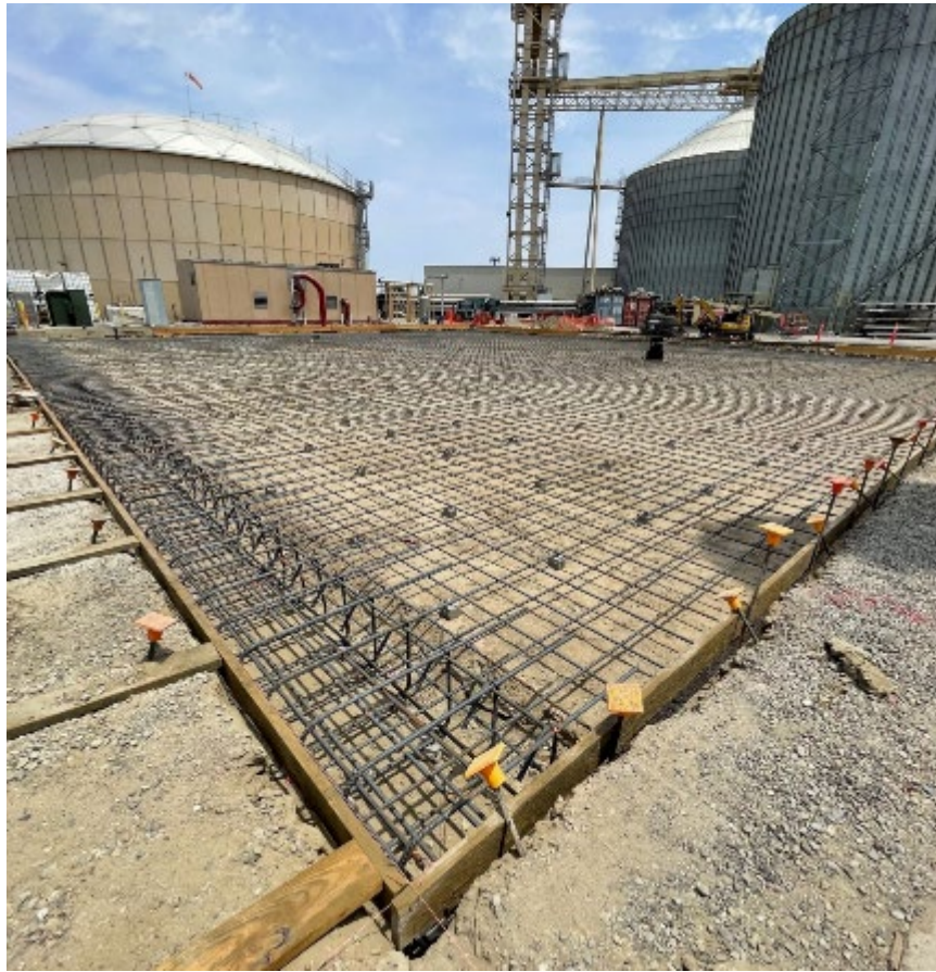
Figure 10: Aemetis Biogas Upgrading Facility Foundation
