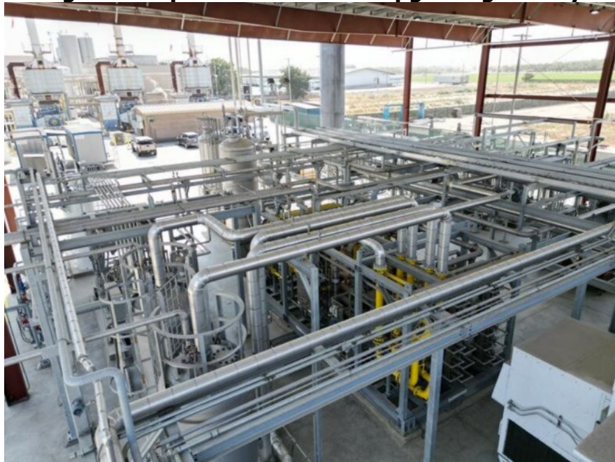
Figure 2:Top View of Aemetis Upgrading Facility
