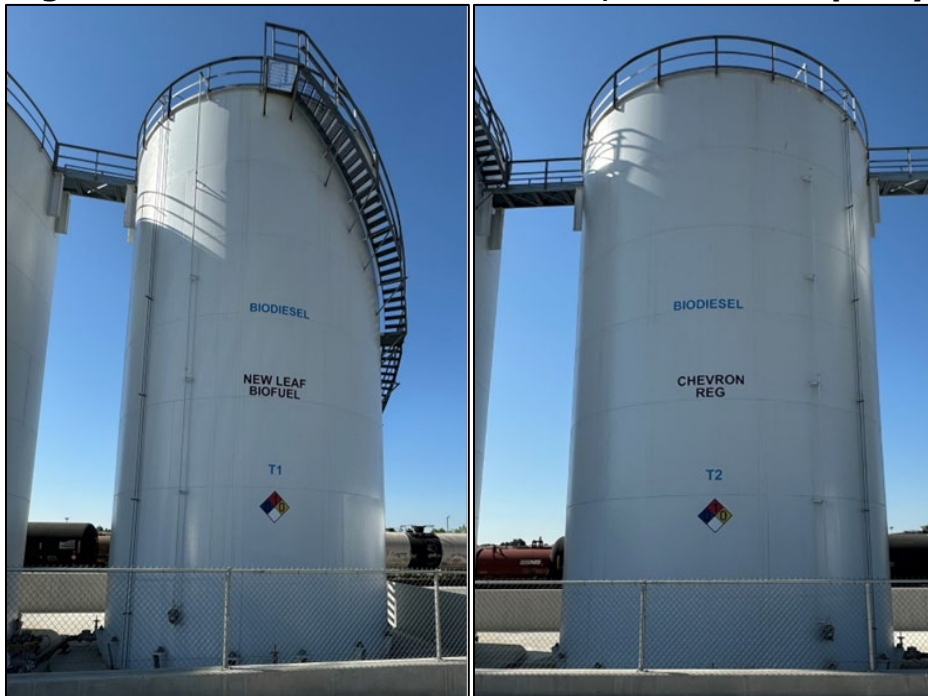
Figure 9: Two Biodiesel Tanks with 8,530 Barrel Capacity
