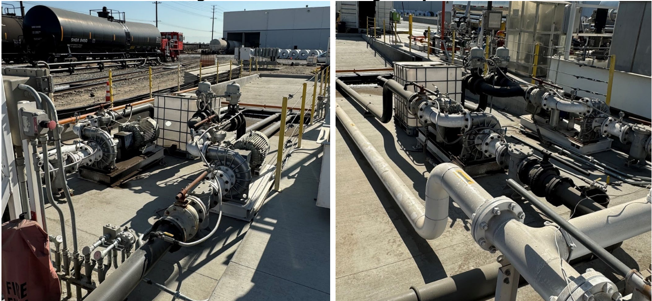
Figure 11: Rail Unloading Pump Skids
