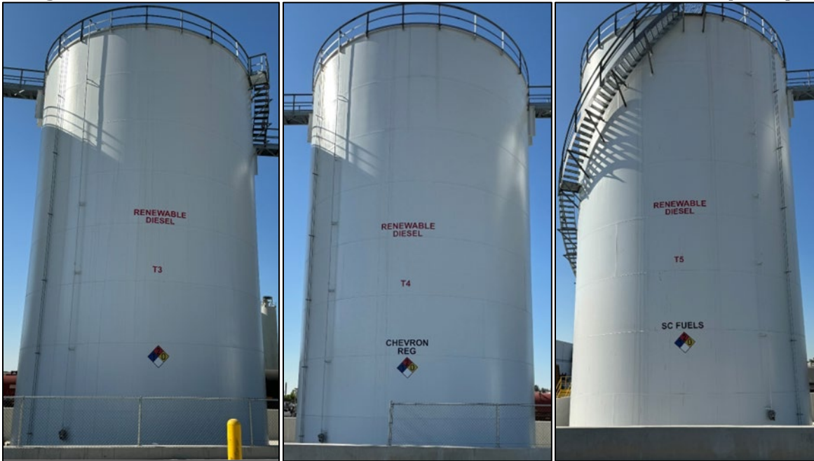
Figure 8: Three Renewable Diesel Tanks with 13,610 Barrel Capacity
