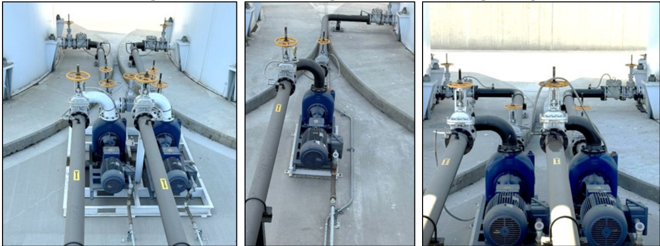
Figure 10: Tank Discharge to Truck Loading Pumps
