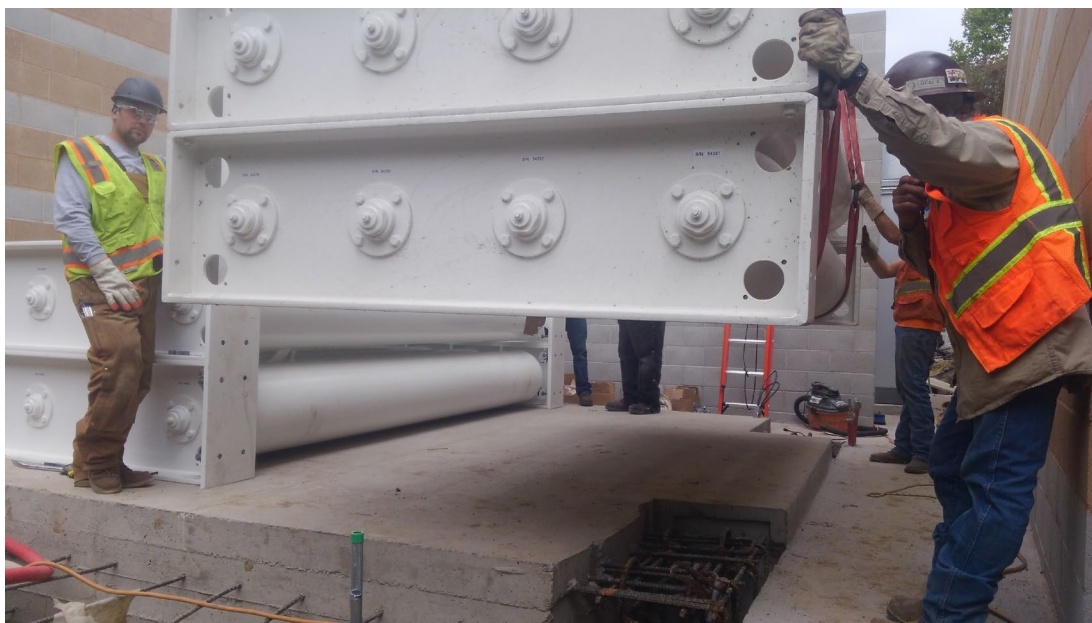
Figure 4: Field Assembly of Storage Module (above); Two Station Modules Under Construction (below)
