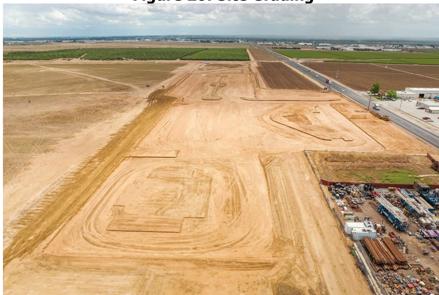
Figure 20: Site Grading
