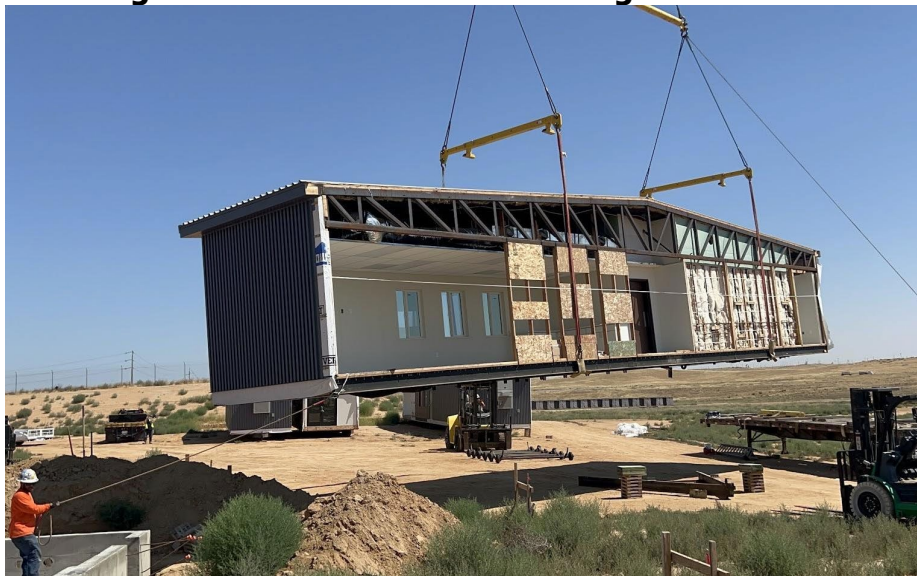
Figure 22: Prefabricated Building Installation
