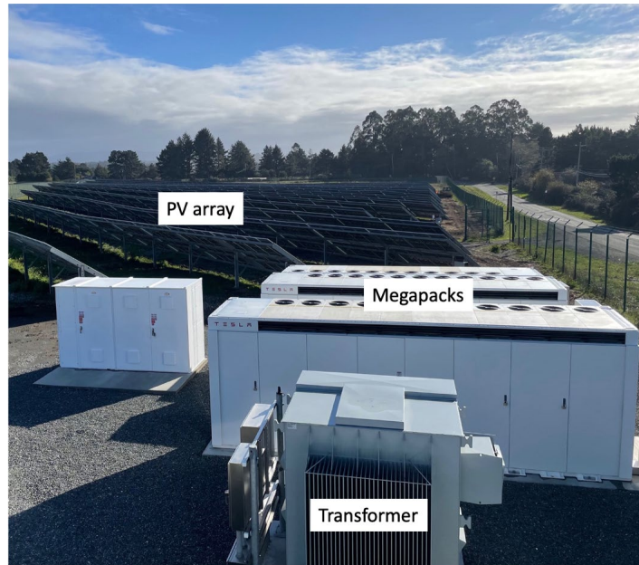
Figure 8: Tesla Megapacks and Transformer
