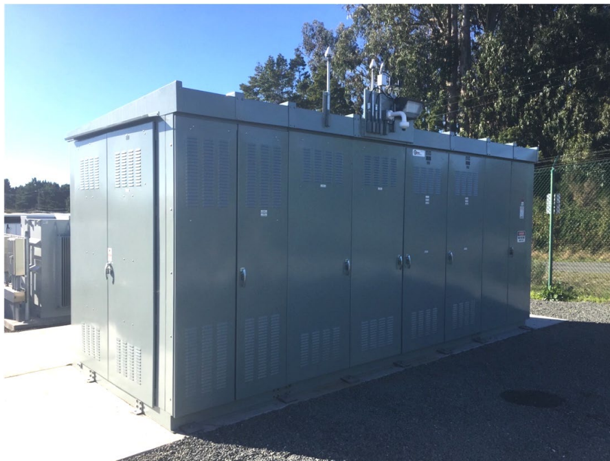
Figure 7: Microgrid Main Switchgear
