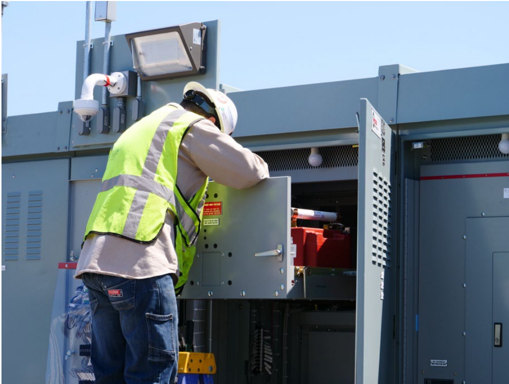
Figure 23: Pre-energization Testing
