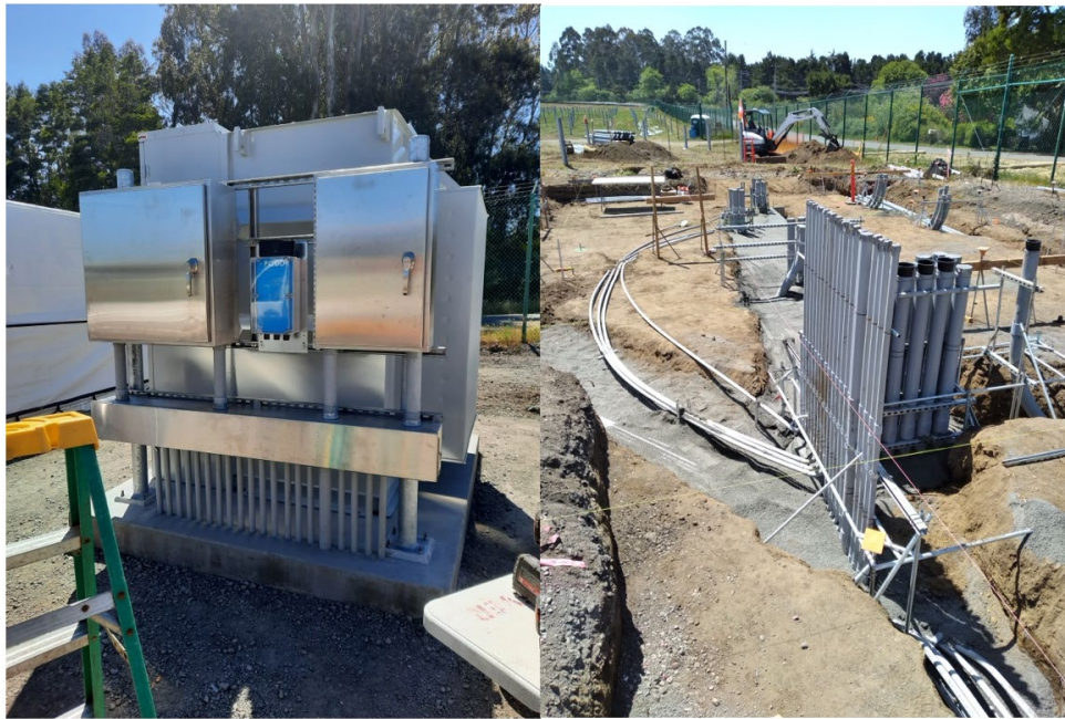
Figure 14: Installation of Transformer and Electrical Conduit
