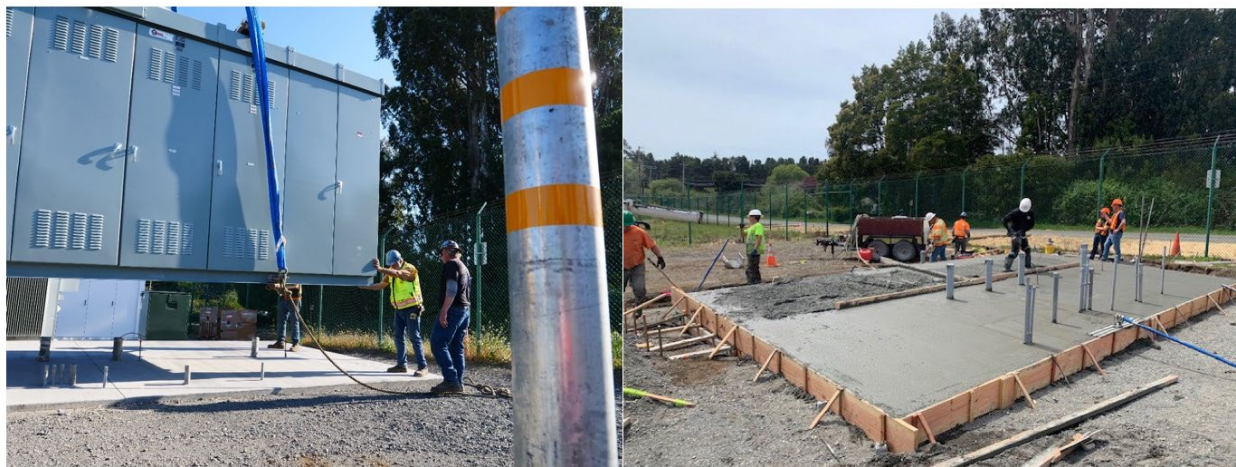
Figure 15: Installation of the Medium Voltage Switchgear
