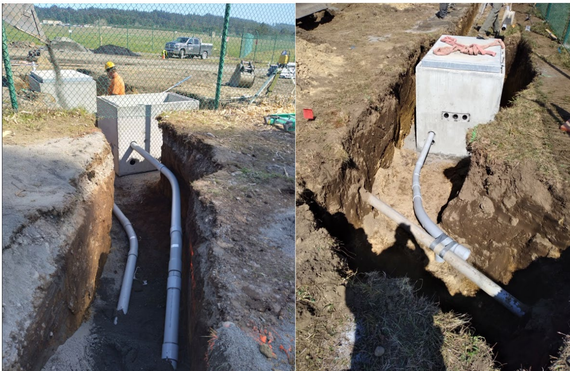
Figure 13: Installation of PG&E and AT&T Underground Service Equipment
