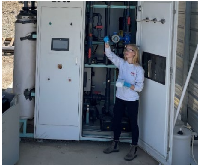
Figure 13: UF Pilot Skid at the Meadowbrook WWTP
