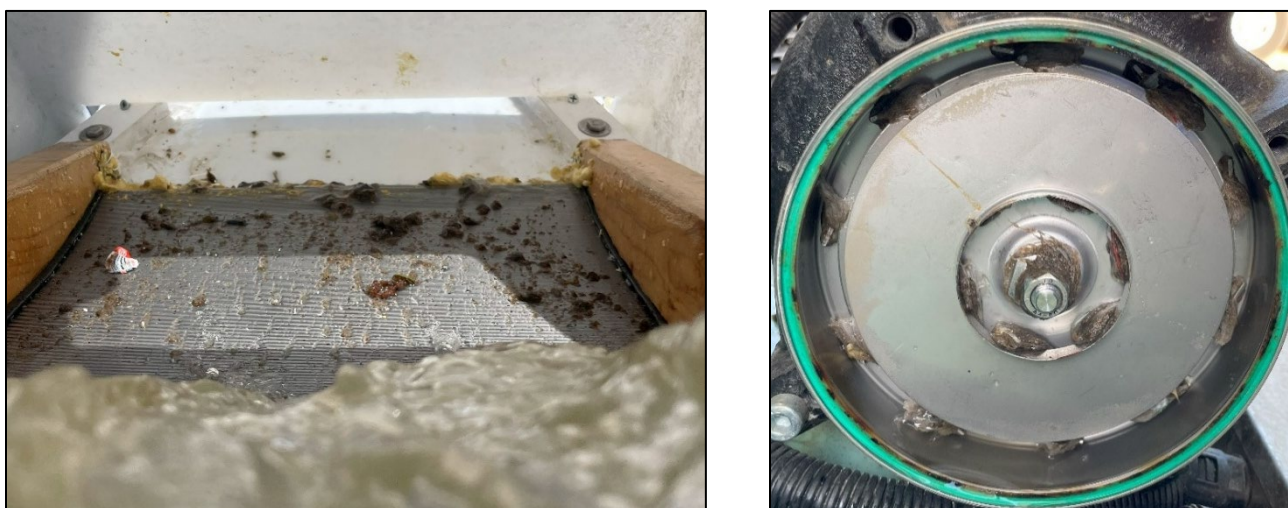
Figure 25: Evidence of Fouling Within the UF Skid Components
