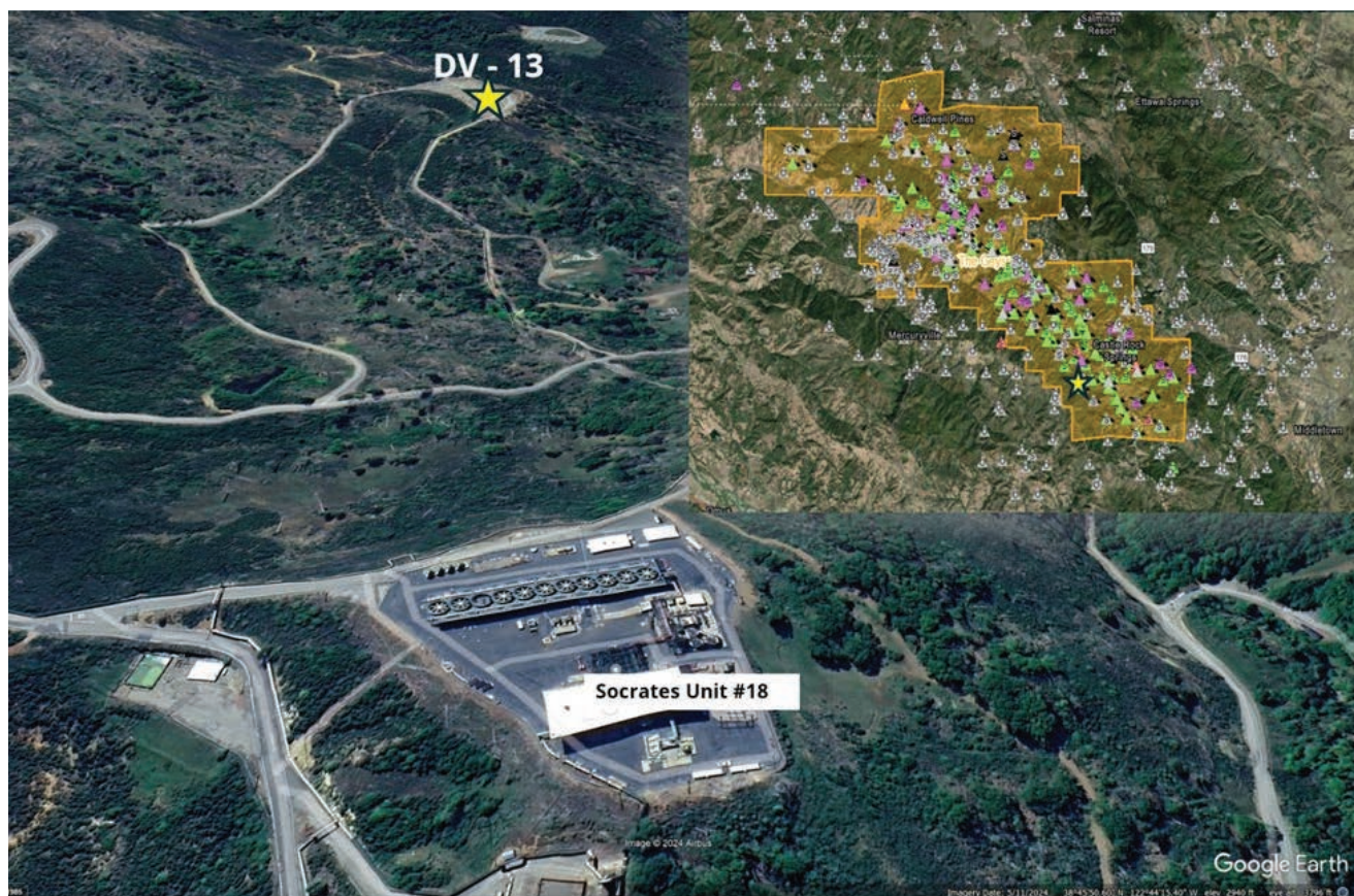
Location of the well DV-13 indicated by the yellow star along with the Socrates Unit 18 power plant. The top right hand corner photo shows all the wells in The Geysers geothermal field and the yellow star on the bottom left of the field indicates the location of the well DV-13.
