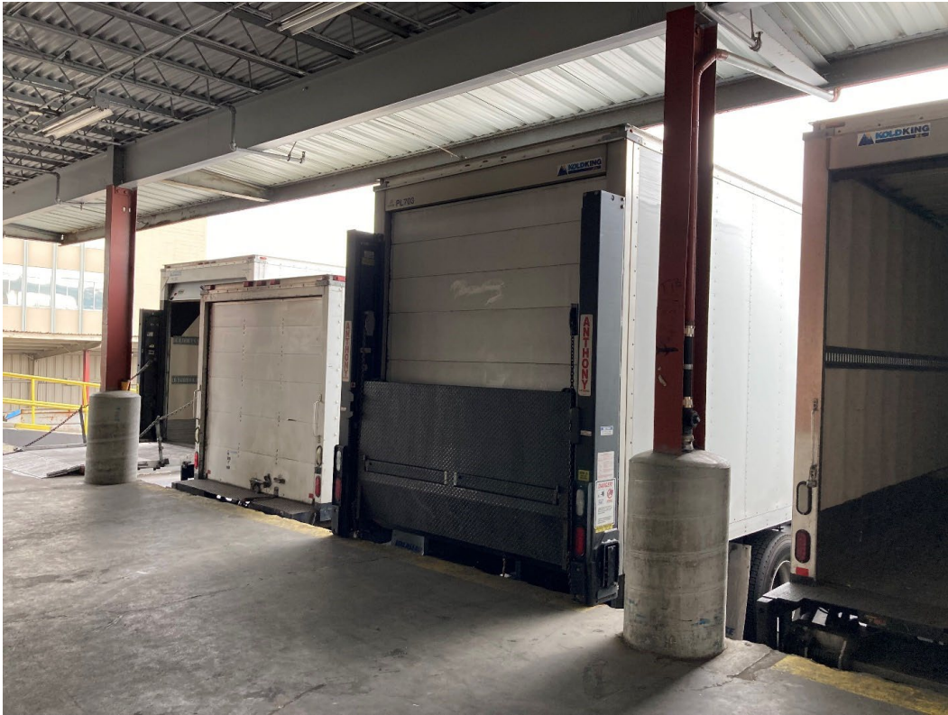
Figure 10: Tenant's loading dock at The SF Market
