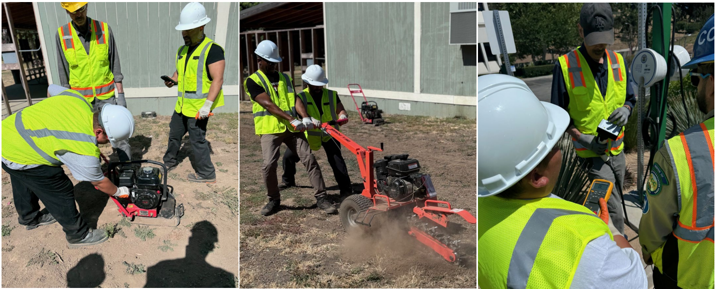
Figure 1. Trainees with Compactor, Trencher, and Testing Meter
