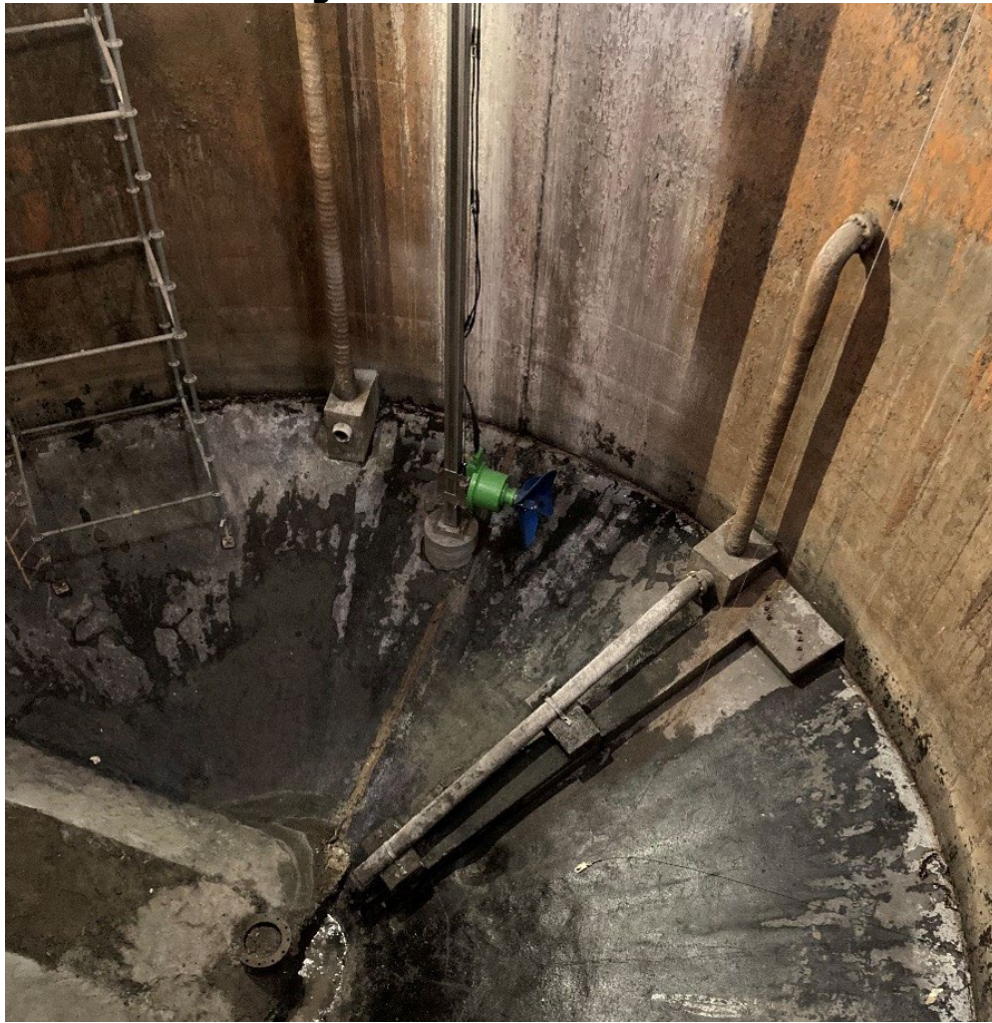
Figure 4. Mixer Installation
