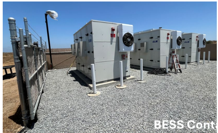
Figure 4: The BESS Switchboard (left) and Containers (right)
