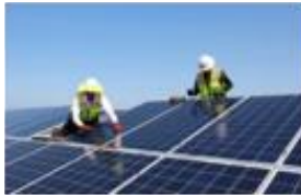
Left: Workers install rooftop solar panels
