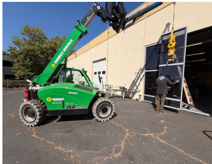
Figure 13: Installation of the BIPV Facade at NEXT Headquarters
