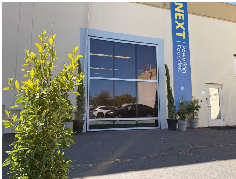
Figure 14: External View of the Completed Facade
