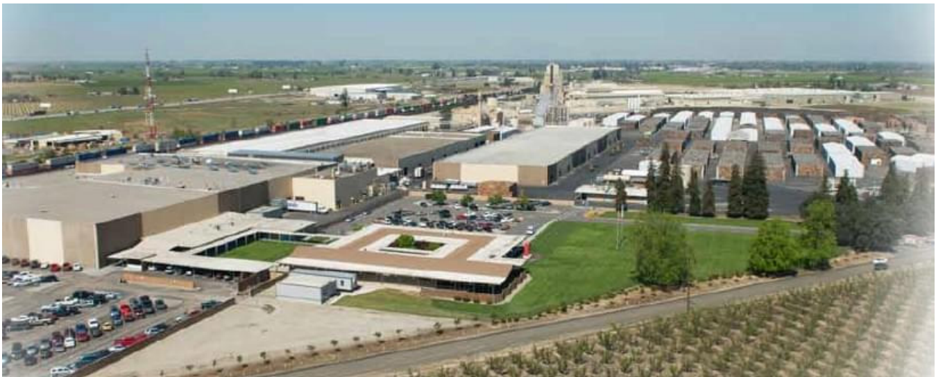
Figure 1: Overview of the Sun-Maid Kingsburg Facility
