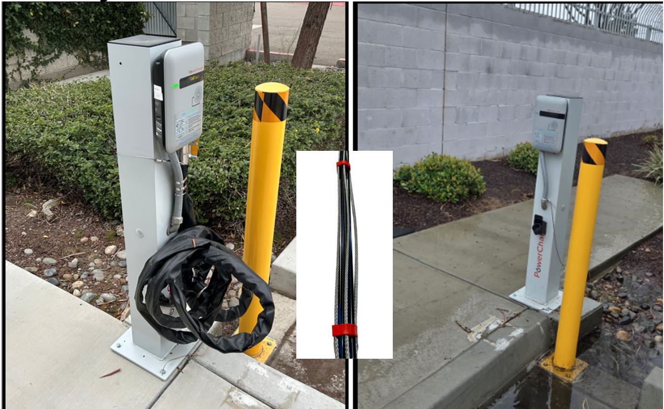
Figure 6: Cable Shield Installation for Prevention of Vandalism
