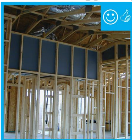
Air barrier installed to unconditioned space
