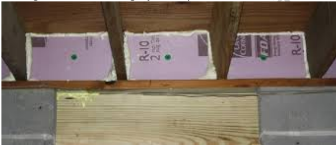
Blocking installed at rim joist/rafter and sealed
