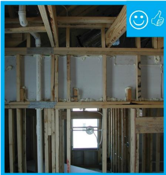
Perimeter blocking installed and sealed
